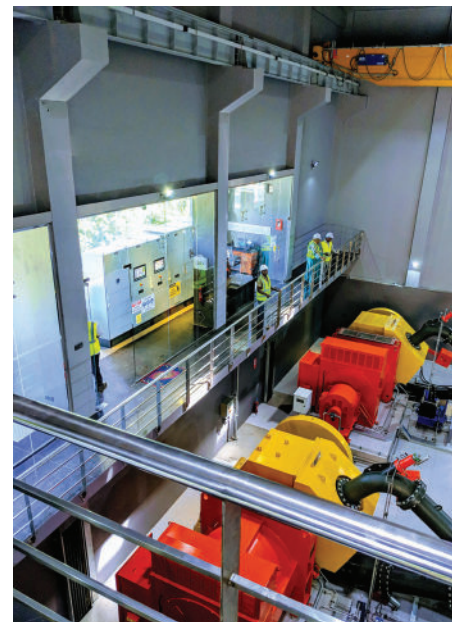
Above: Turbine Generators & Control Room at Lubilia
