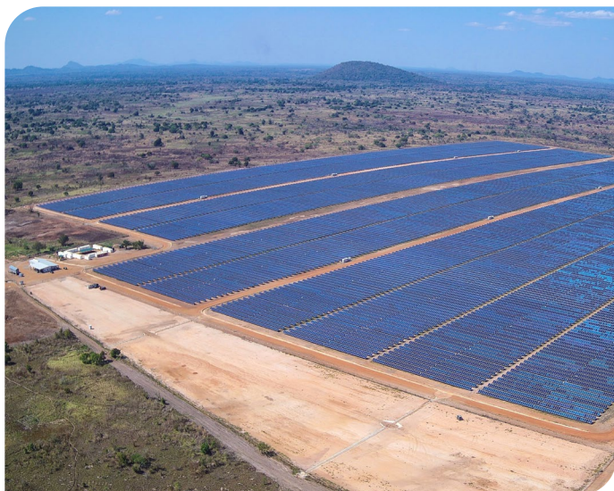
The 40MW Central Solar De Mocuba plant in Mozambique is one of 23 renewable energy plants EAIF has supported to date. Picture courtesy Scatec Solar.
